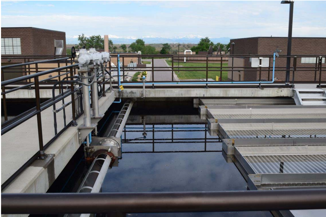
Northern Treatment Plant, taken in 2021
