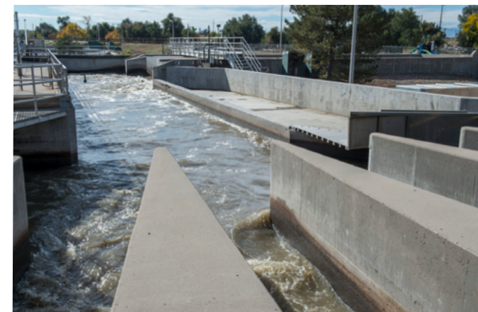
RWHTF influent channels.
