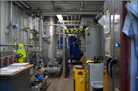
The thermal hydrolysis pretreatment pilot was in a trailer west of the Digester Complex.
